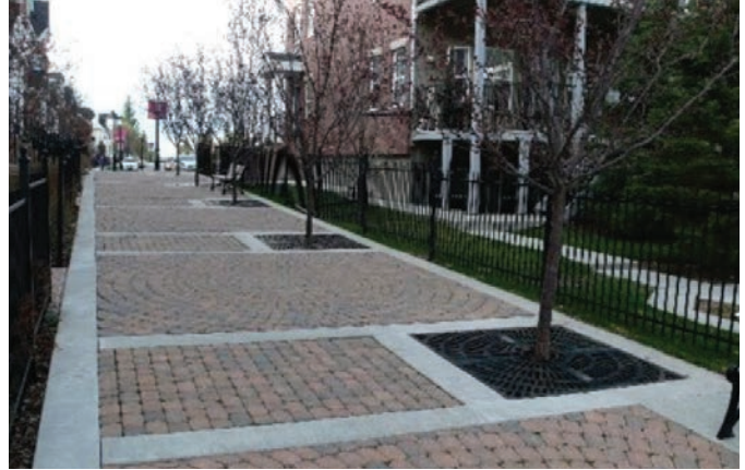
Figure 2.23: Pervious pavers with tree wells
