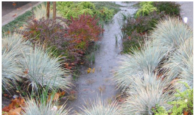
Figure 2.24: Bioswale filters stormwater
