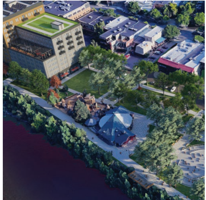
Figure 2.68: Potential mixed-use building with parking and community facility in Caras Park (Long-Term Scenario)
