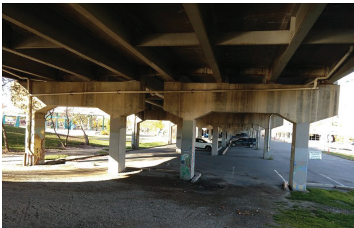
Figure 2.50: Higgins Avenue underpass existing condition
