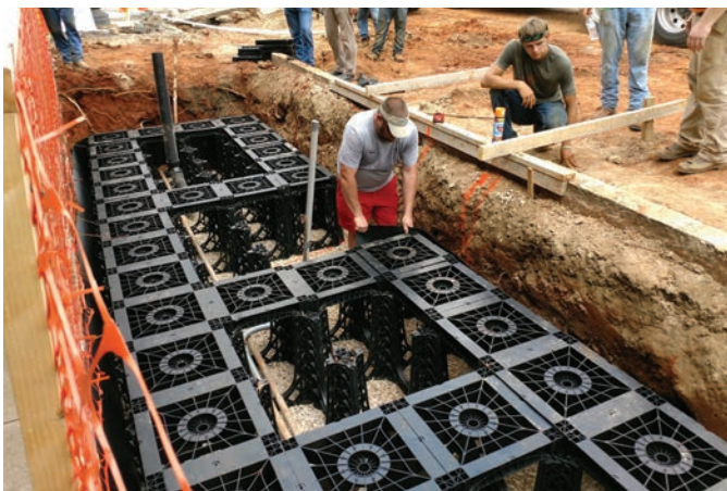
Figure 2.22: Tree wells with Soil Cells
