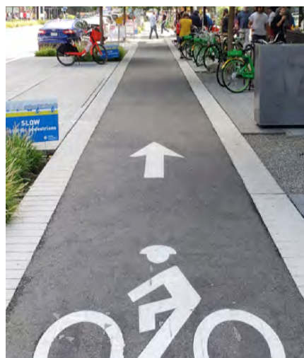
Images of three types of bicycle lanes – traditional striped lane (top), buffered lane (middle), and separated lane (bottom)
