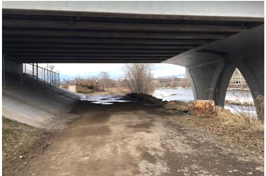
Existing conditions of Orange Street Underpass
