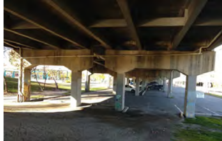
Higgins Avenue Underpass Existing Conditions
