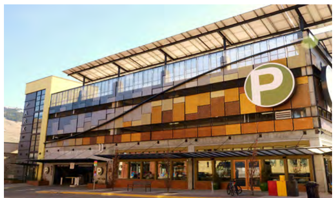
Park Place Parking Garage
