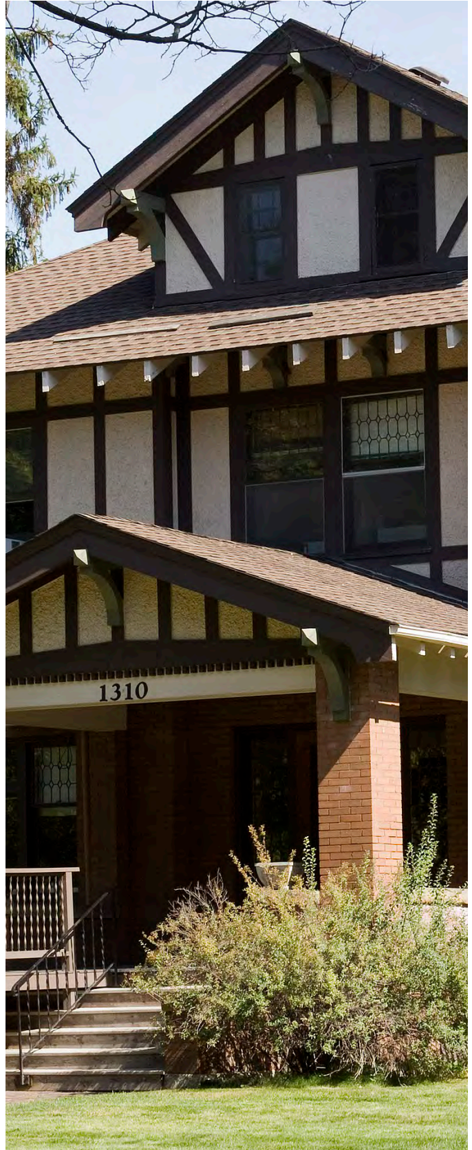
Fred T. Sterling House (1912) - 1310 Gerald Avenue Added to the National Historic Register in 1983.
