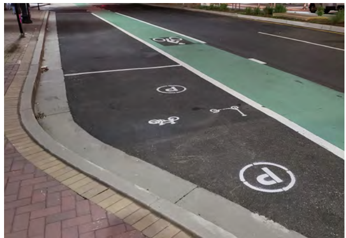
Designated space along the curb for parking dockless micro-mobility vehicles in previously unused space
