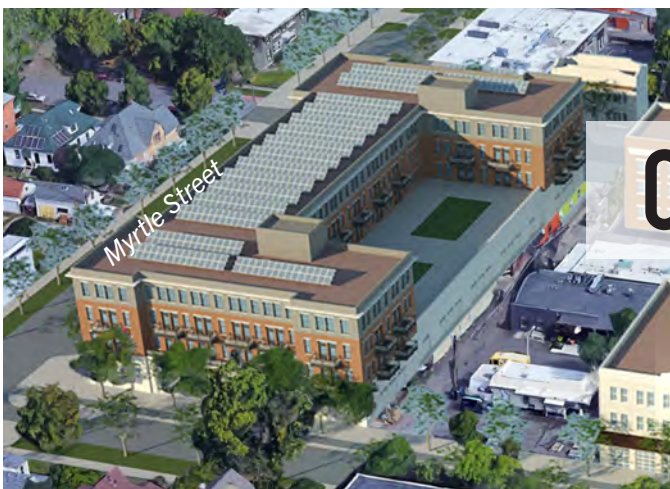
Underground parking with mixed-use development
