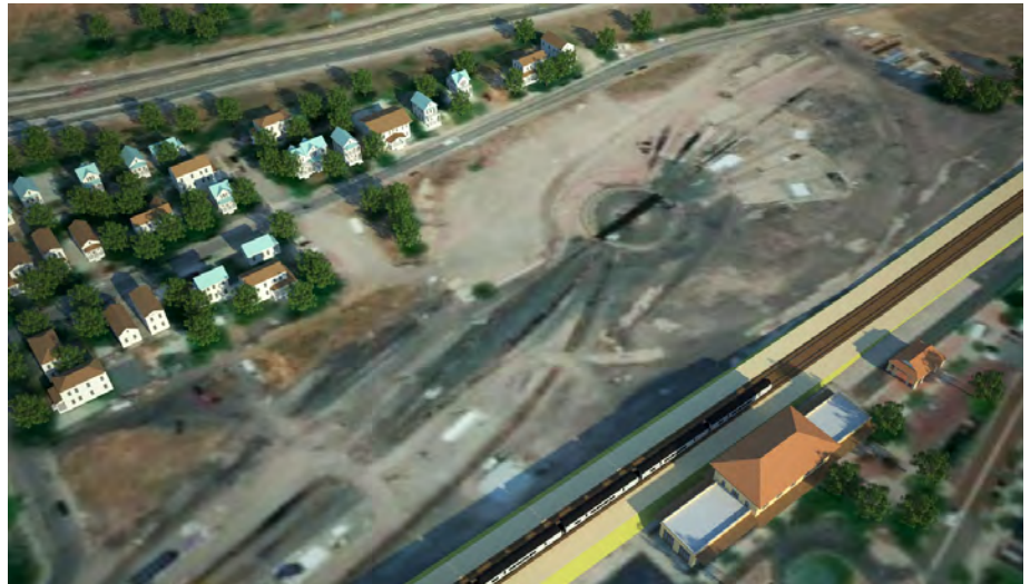
Railyard existing conditions showing switchyard
