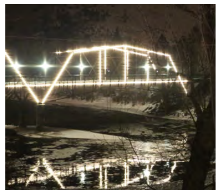
Van Buren Street footbridge light installation
