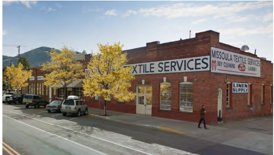
Existing Missoula Textile Services Building on E Spruce and N Pattee Street
