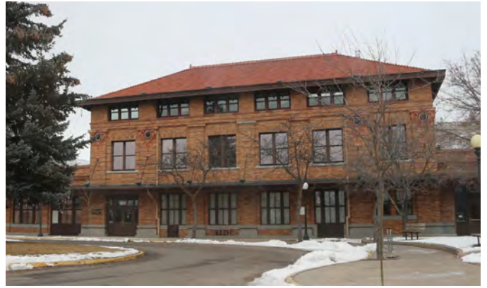
Northern Pacific Railroad Depot - 100 Railroad Street
