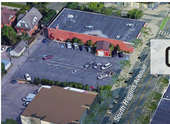
All parking remains on-site at the Senior Center
