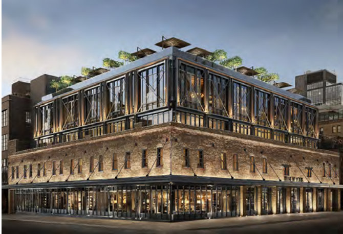
2-Story Commercial Addition in Manhattan by Backen & Gillam Architects
