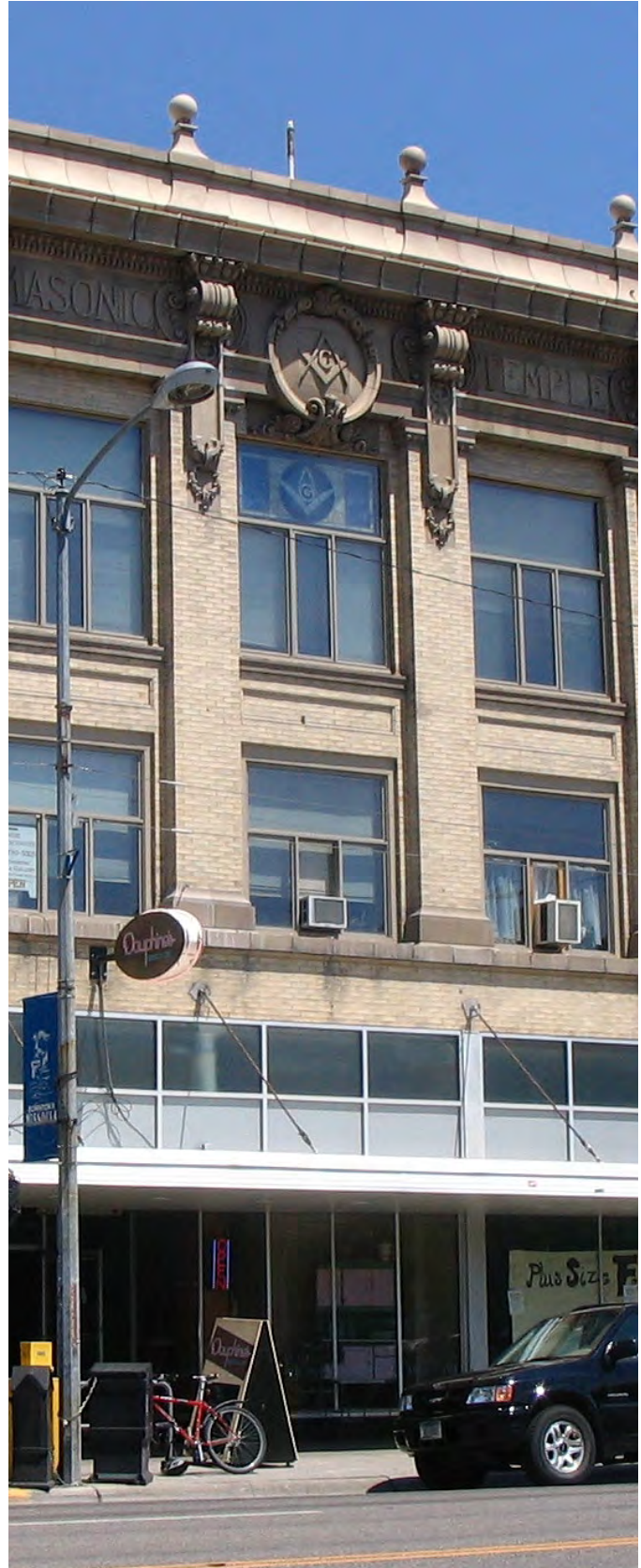
Masonic Lodge (1909) - 120-136 East Broadway Avenue. Added to the National Historic Register in 1990.
