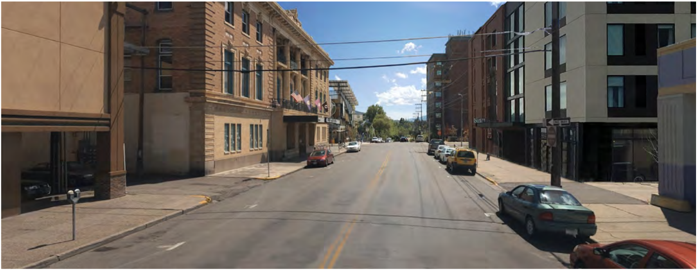
Pattee Street Between Front and Main streets looking south - Existing Condition
